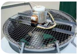
• A fan's airflow has a linear relationship with fan speed, but a fan's power consumption has a cubic relationship with fan speed 9
